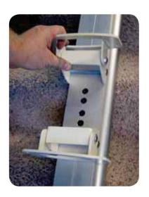
clearance, move the rail and bracket forward towards the nose of the tread. Once the clearance is 2", tighten all bracket nuts to hold the rail in position.
